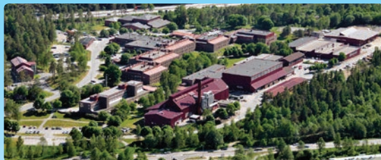
SP Technical Research Institute of Sweden's site in Borås
