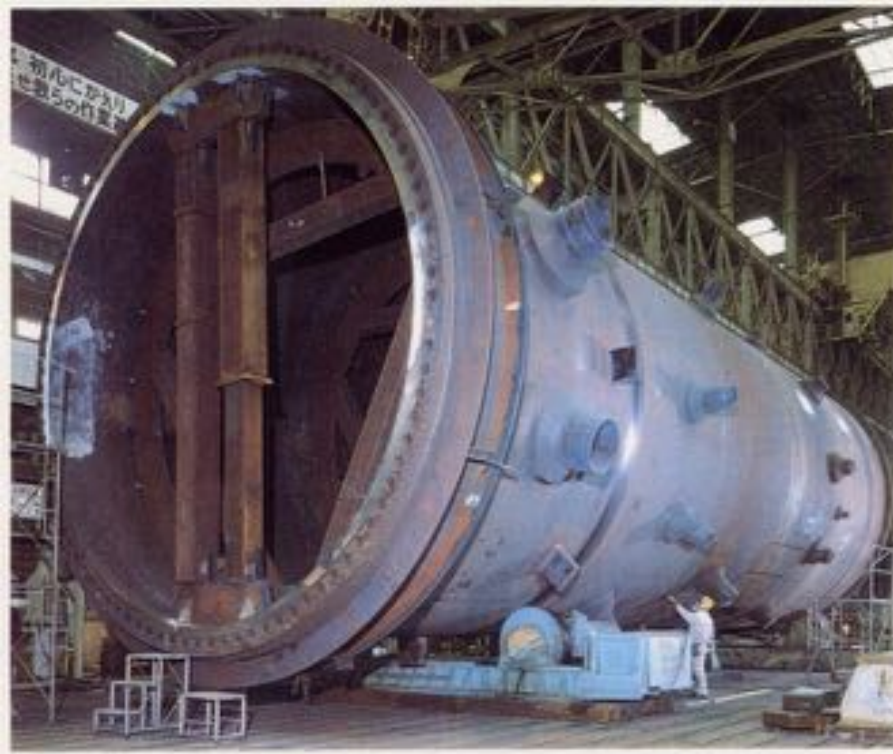
Circumferential welding of a reactor vessel by submerged arc welding
