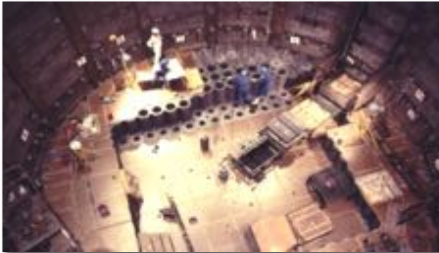
Heysham 2 (during construction)
