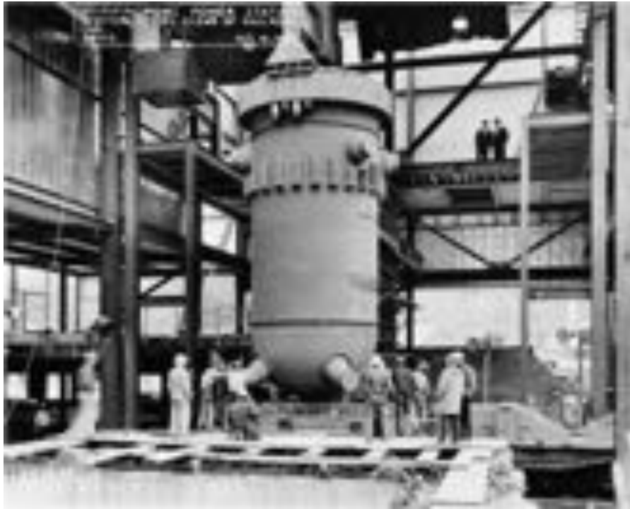
Shippingport during construction
