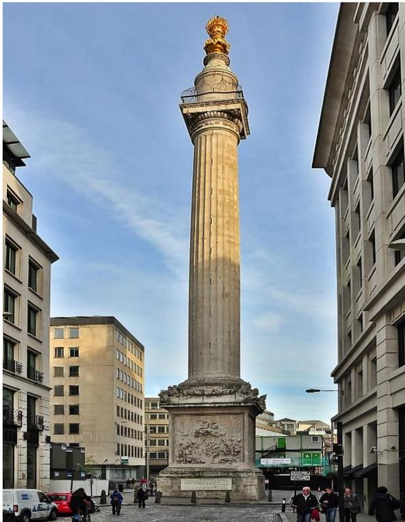
**Fig.1:** The Monument, London. This structure consists of a simple stone tube of height about 70m, with no windows and a basement laboratory. There is a clear aperture from the basement, up the centre of the internal spiral staircase, to the top.
